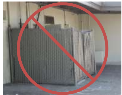
Fig 13: Prohibited chain link fence
