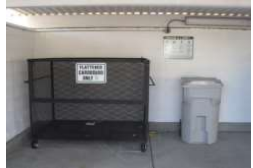
Figure 16: Signage and lighting within trash enclosure
