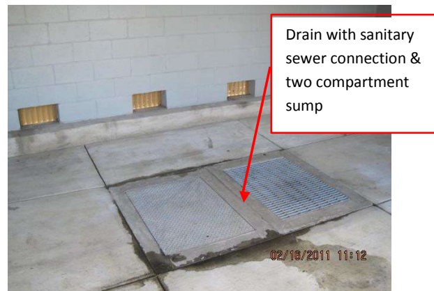
Figure 5: Sanitary connection with sump
