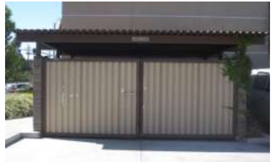
Figure 14: Metal Trash Enclosure Gates
