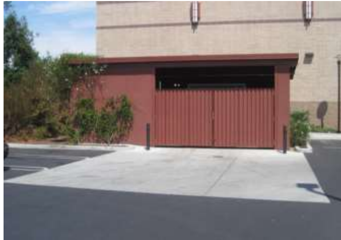
Figure 22: Trash enclosure for compactor
