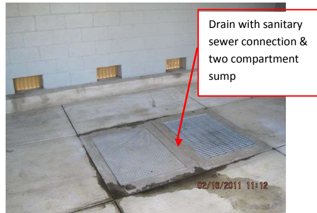
Figure 5: Sanitary connection with sump
