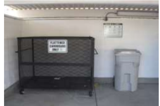
Figure 16: Signage and lighting within trash enclosure
