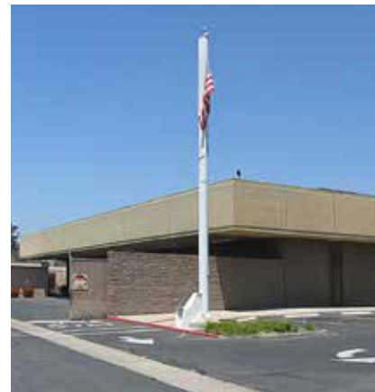
Copyright © 1997-2016 CellTowerPhotos.com. Used with permission.
