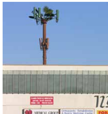
Copyright © 1997-2016 CellTowerPhotos.com. Used with permission.
