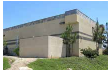
Copyright © 1997-2016 CellTowerPhotos.com. Used with permission.
